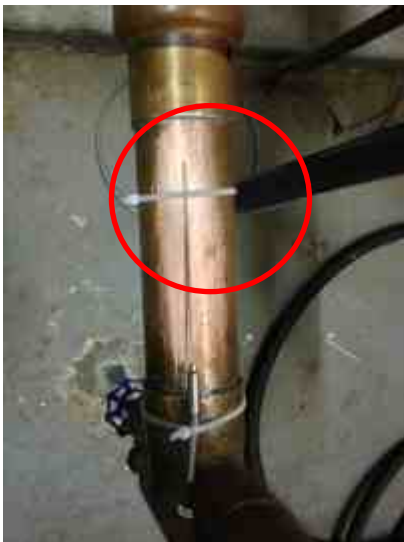
Figure 14. Supply water temperature ( T_S , left), recirculation loop temperature ( T_R , right)
