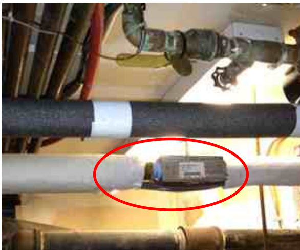
Figure 17. Flow sensor (left), and OPTO 22 data logger (right)
