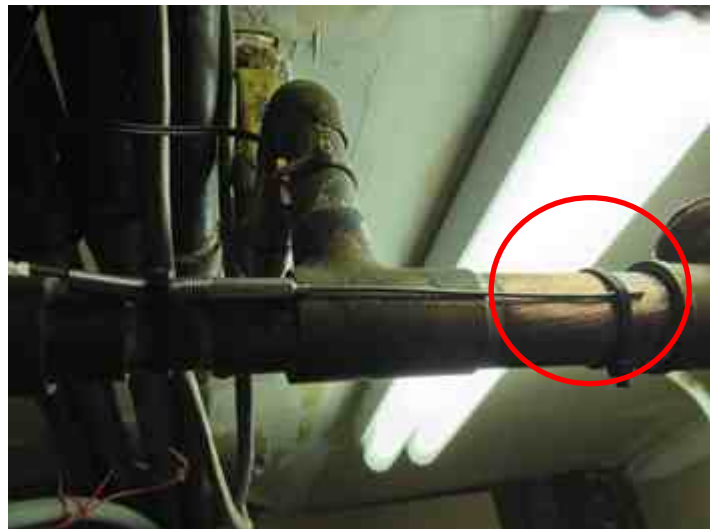
Figure 14. Supply water temperature ( T_S , left), recirculation loop temperature ( T_R , right)
