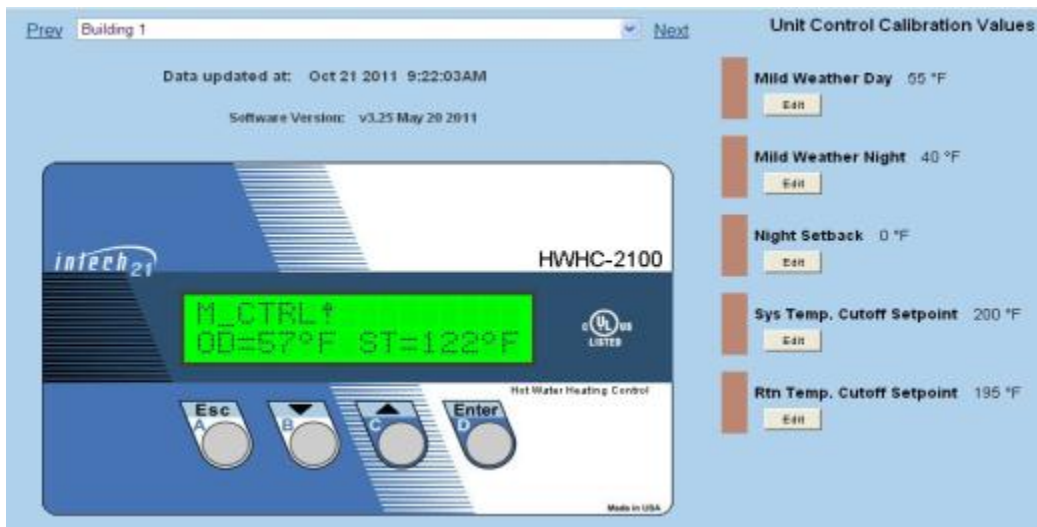
Figure 6. Controller Web interface
