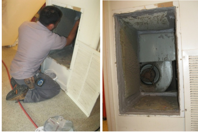
Figure 6. Applying mastic inside metal return plenum 6
