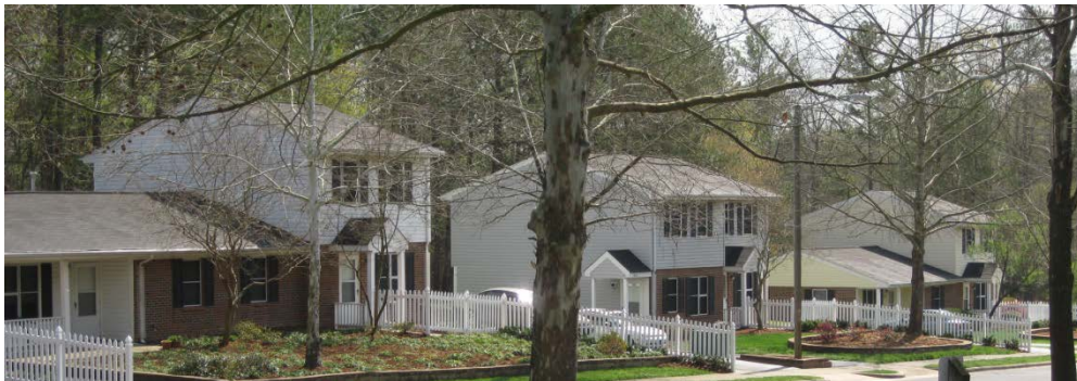
Figure 1. One- and two-story attached homes at TP
