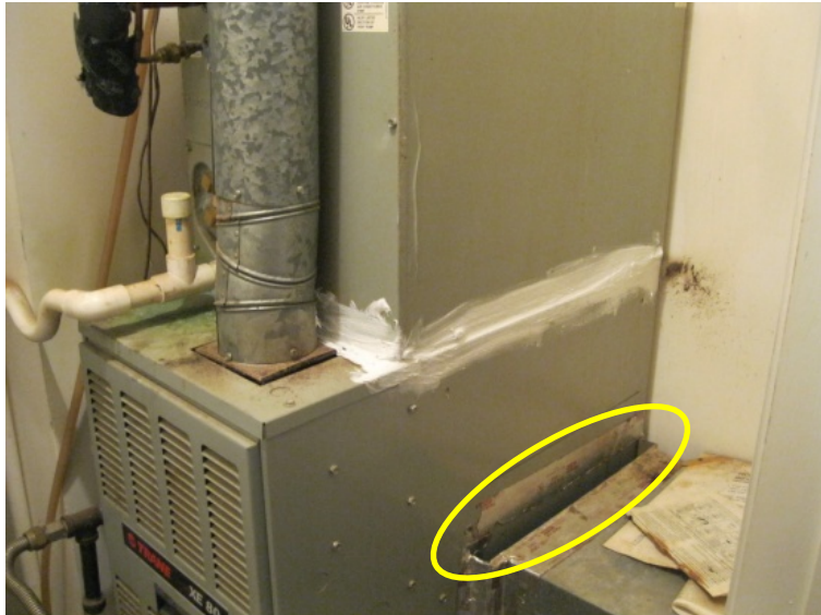
Figure 11. Filter slot at BVC one-story unit
