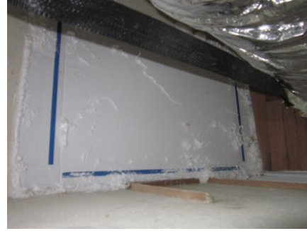
Figure 12. After: Opening in wall above dropped ceiling patched and sealed
