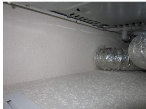
Figure 10. After: Sealed wall above dropped ceiling
