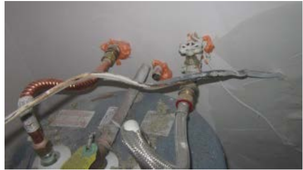
Figure 20. After: Water heater pipe penetrations sealed with foam
