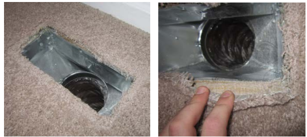
Figure 6. After: Boots sealed to subfloor
