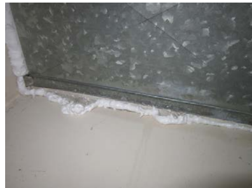
Figure 24. After: Gap around supply duct sealed with foam
