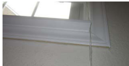
Figure 14. After: Window sill sealed to wall with caulk
