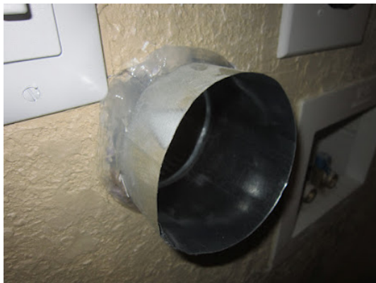
Figure 23. After: Dryer exhaust duct sealed to wall with caulk
