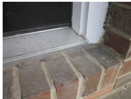
Figure 22. After: New door sweep and sill sealed to brick
