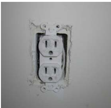
Figure 21. After: Outlet sealed to wallboard around perimeter
