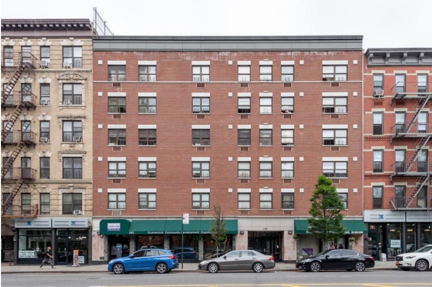
Figure 1 439 West 125 th Street
